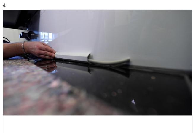
**5** Step by step, the bath is designed to work well for older people with physical limitations. When installing the shower toilet, the TOTO-trained technicians professionally adjust the fitting panel to meet the available space. The water and power connections are integrated in the back of this panel. This makes it possible to install WASHLET™ without doing any renovation work. Photo: TOTO
